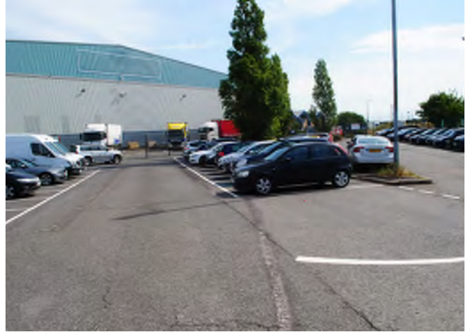
Location 10: Entrance to Unit 1
