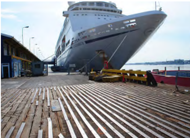
Location 1: Looking E along passenger Landing Stage
