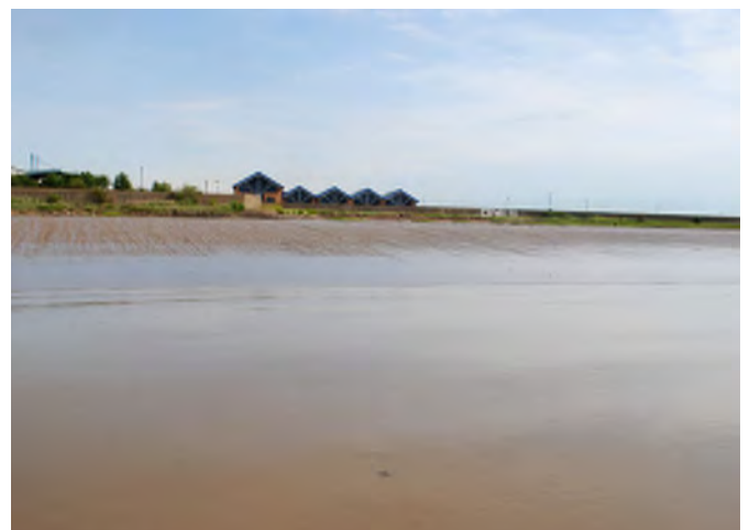
Location 2: Looking N towards River Wall
