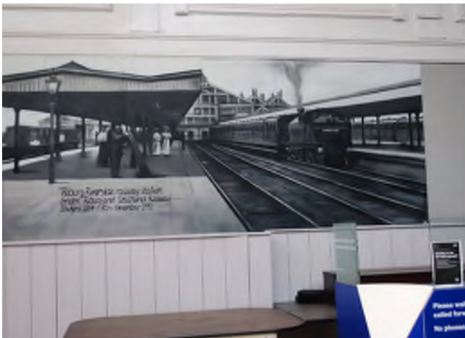
Location 12: Inside Railway Station – photo recording station use
