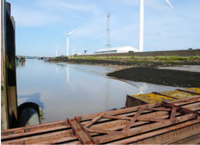
Location 1: Looking W. River Wall to right. Floating pontoon to left
