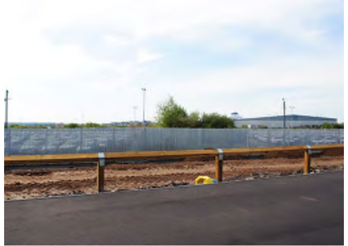
Location 5: Looking S across car storage at D Compound swale visible - from new road
