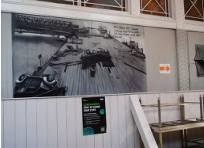
Location 12: Inside Railway Station – photo recording bomb damage
