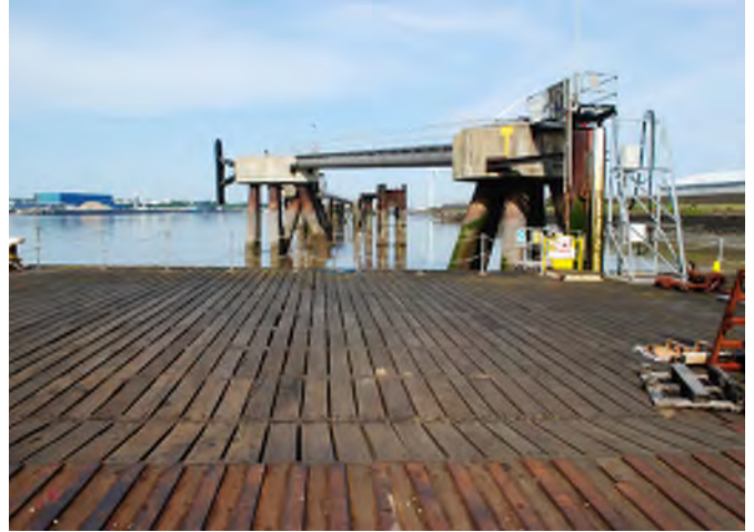
Location 1: Looking W along floating "pontoon ducks"
