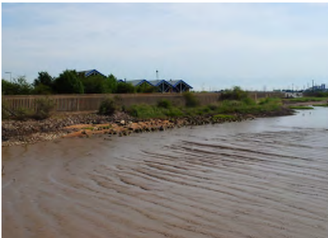
Location 3: Looking NE towards River Wall
