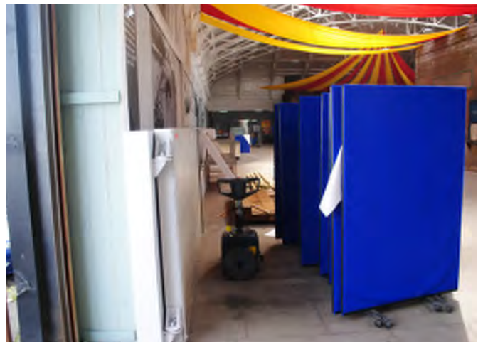
Location 12: Inside Railway Station – flood defence barrier (white walling)
